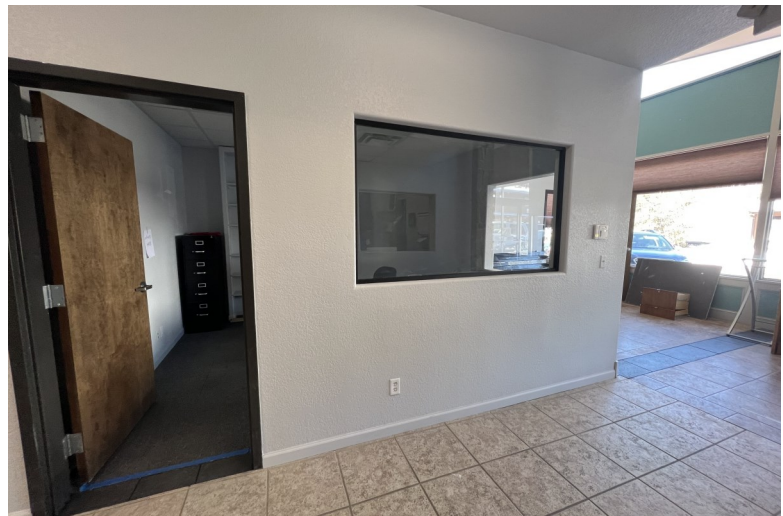
The new front desk reception in progress!
