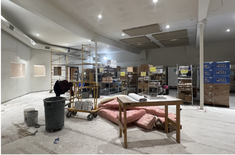
The new food pantry in progress! EEEK!
